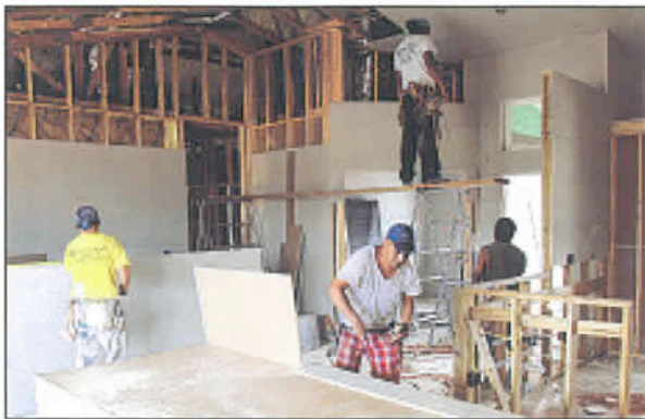
Crews work to construct the green home.
